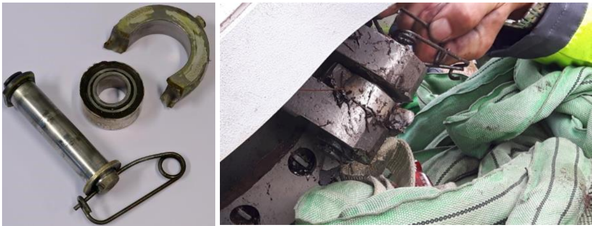
Figure 56: Upper forward suspension bar, part of the mounting lug, the bearing, the clevis pin (with only one of the two safety pins) and the safety pins. Here shown both as found at the rotor mast (right photo) and dismantled (left photo). Photo: AIBN
